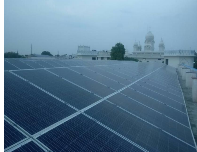
100 KWp off grid plant + 27 KWp Solar Pumping system
